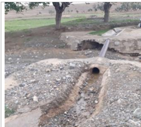
Picture 3.42: Watercourse Damaged due to Heavy Rains and Floods in Pishin
